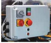
Control box for a 2 speed abrasive belt machine. With speed control switch, on/off push buttons, isolator switch,emergency stop and two indicator lamps.
