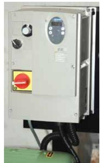
A Telemecanique Altivar 31 inverter. Programmable and with overload protection. This is the standard inverter we use unless requested otherwise.
