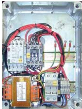
A 24 V control unit. Top from left: Overload relay, main motor on/off contactor, Bottom from left: Transformer, fuses, terminal block.
